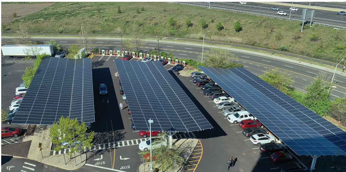
By pedrik - Parking under Solar Canopy, CC BY 2.0, https://commons.wikimedia.org/w/index.php?curid=137148049
